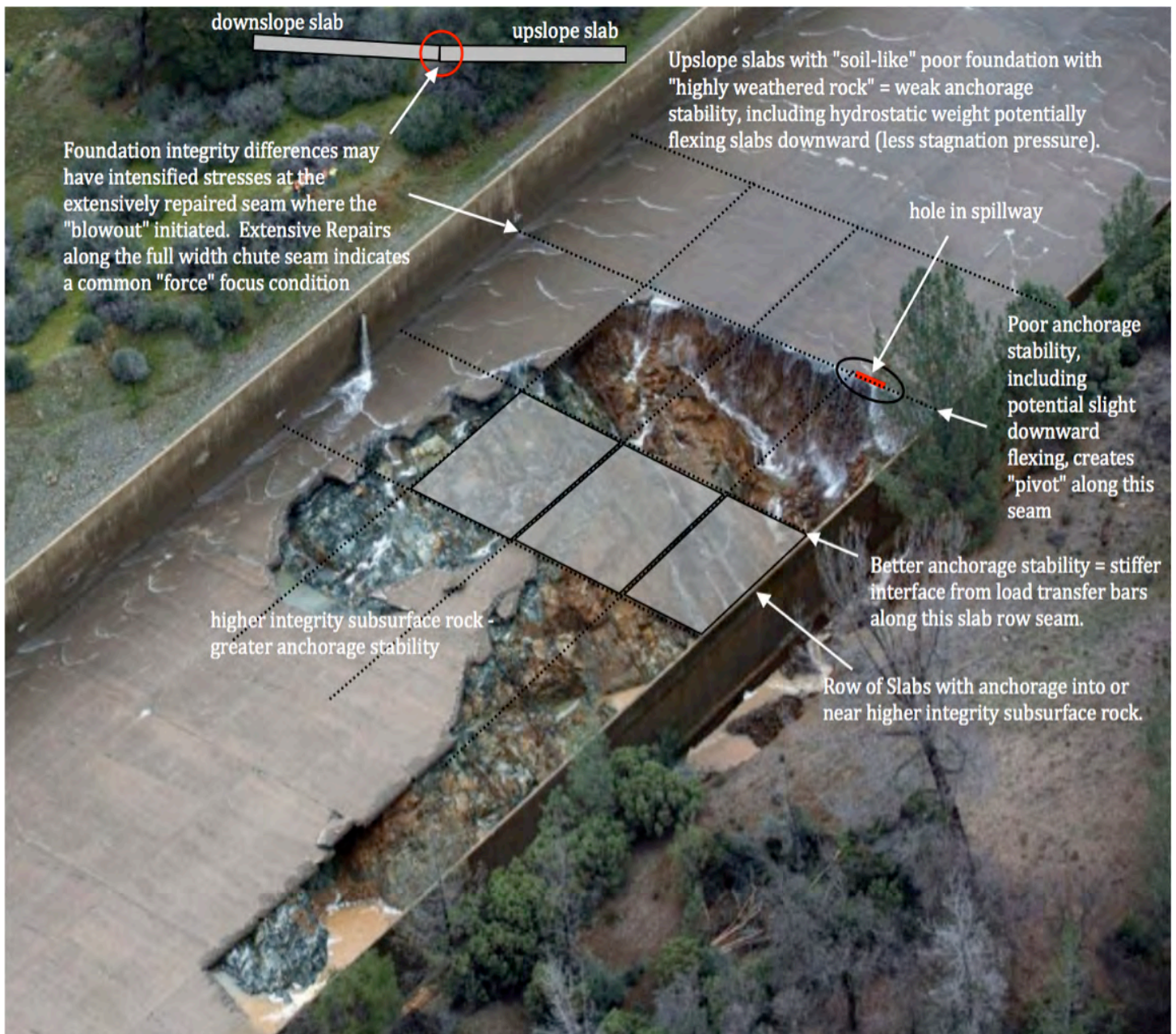
Fig. B.11. Blowout Failure slabs located at a transition zone of higher integrity anchorage stability slabs versus slabs emplaced on poor anchorage stability based slabs above "soil-like" erodible foundation material (incompetent rock).
